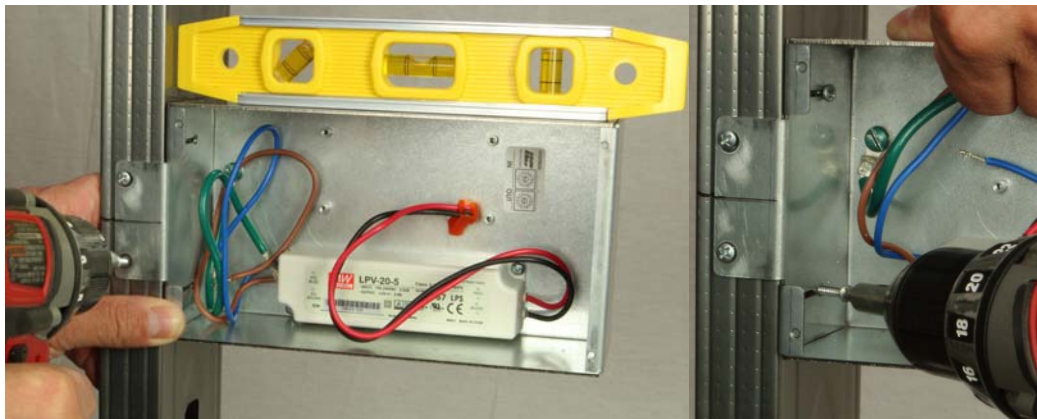
Figure 3 Securing the Enclosure
