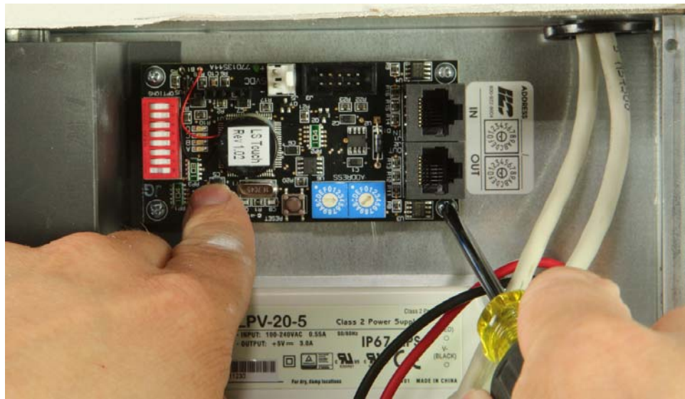
Figure 9 Installing Electronics
