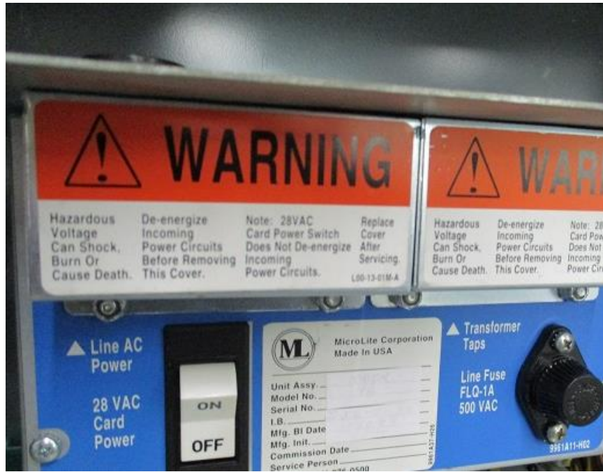
Figure 3 Existing Power Transformer Enclosure
