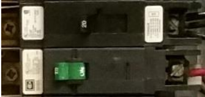
Figure 2 Standard Breaker(above) GHBS Controllable Breaker(below)
