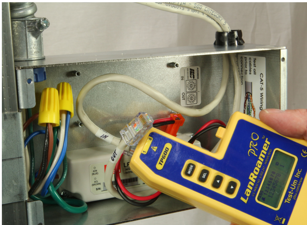
Figure 5 Testing the CAT-5 data cable
