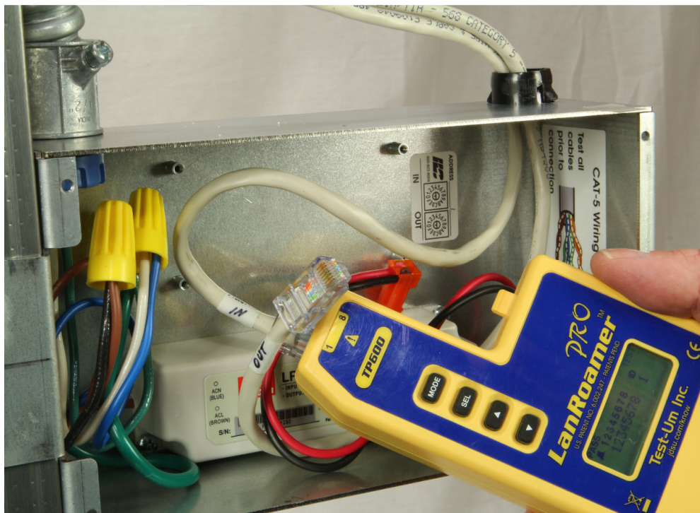
Figure 5 Testing the CAT-5 data cable
