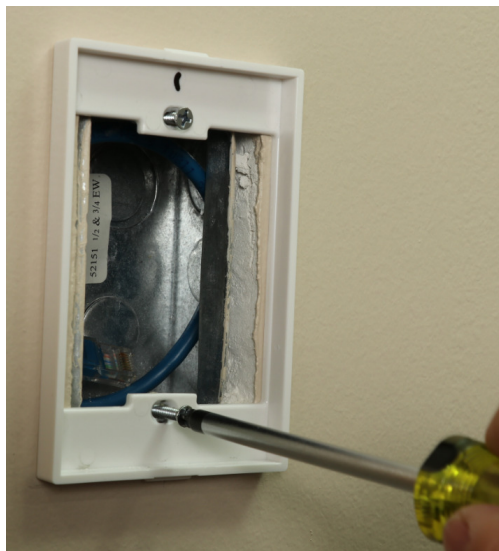
Figure 1 3.5" TSS Mounting Bracket
